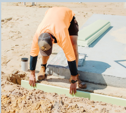
Installed below finished ground level on a standard WA strip footing.
